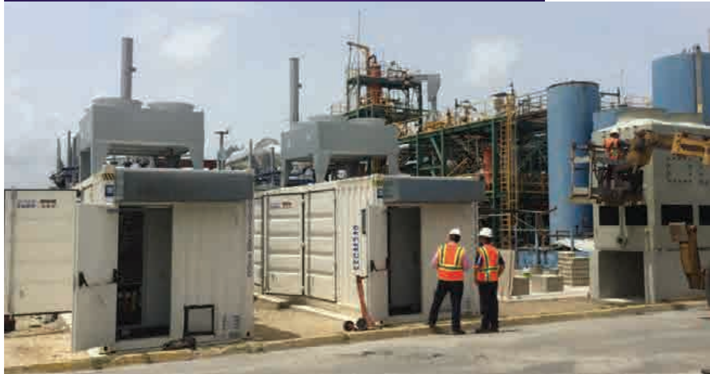
Olefin food industry plant, two containerized SGE-24SM engines.
