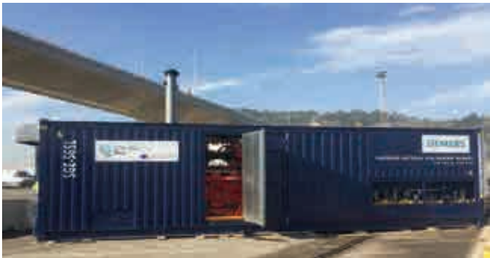
Containerized 56SL genset for harbour use.
